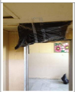
Figure 41: plastic bags fixed to the sealing to prevent water leaks
